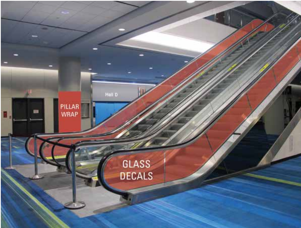
Example 5. Glass decals, pillar wraps Exhibit Hall D escalators up to Level 700
